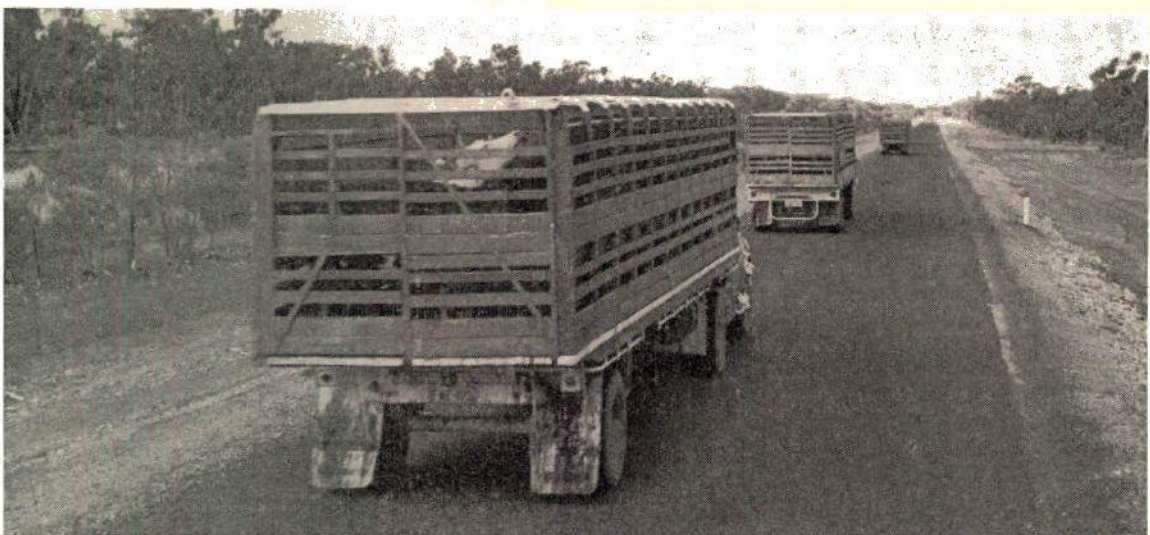
Reconstructed and bitumen-surfaced pavement on the Mitchell Highway 46 miles south of Bourke
