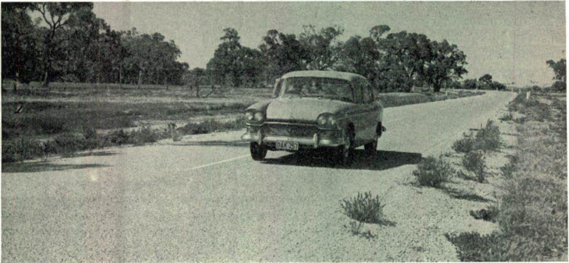
The Wentworth-Mungindi Trunk Road 11 miles north of Wentworth following reconstruction and bitumen surfacing by Wentworth Shire Council
