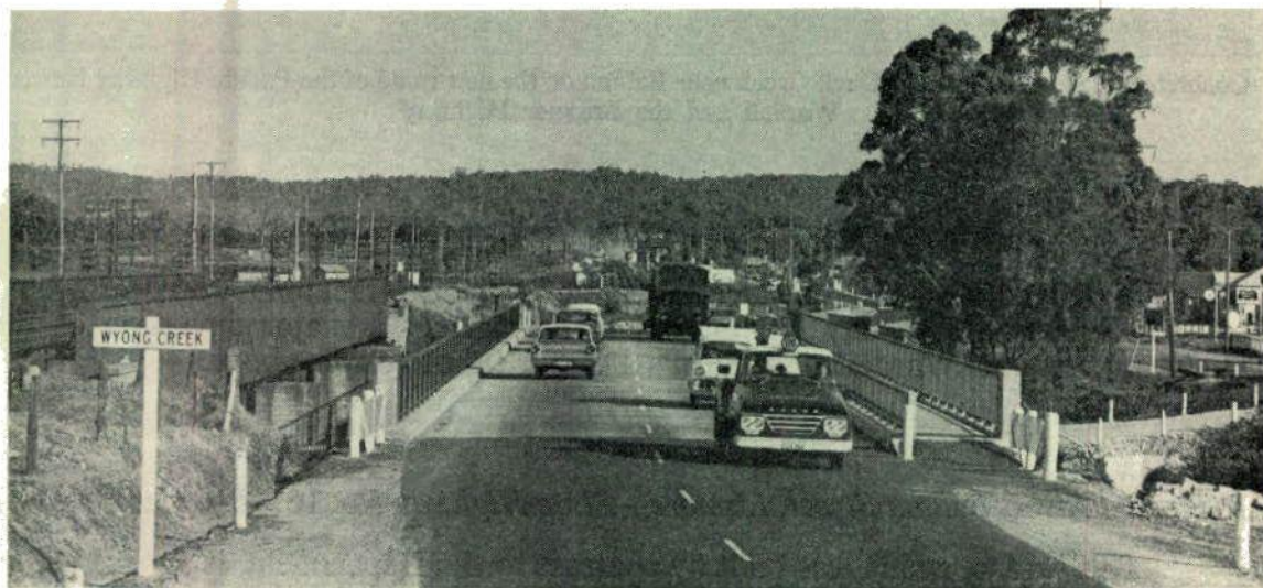
Dissused railway bridge converted for road traffic on the Pacific Highway at Wyong
