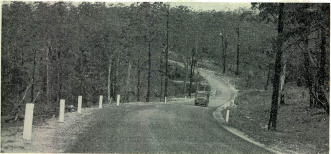
Reconstructed and bitumen-surfaced pavement on the Jenolan Caves Main Road, 14 miles south of the Great Western Highway
