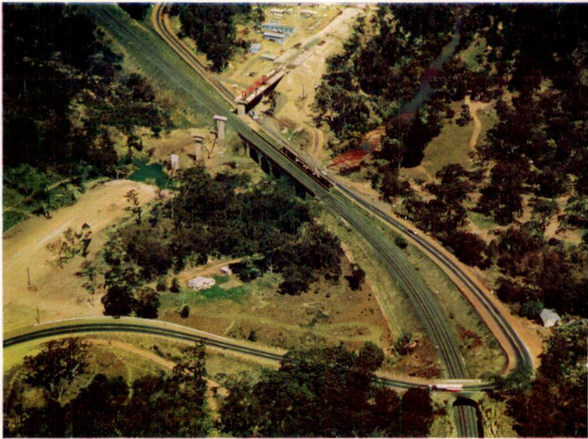
An aerial view of work in progress on the construction of a high level bridge over the main southern railway line and adjacent Bargo River on the Hume Highway (State Highway No. 2), three miles north of Bargo. This work will eliminate the last remaining single lane bridge on the Hume Highway as well as providing much improved alignment on this section of the road.
