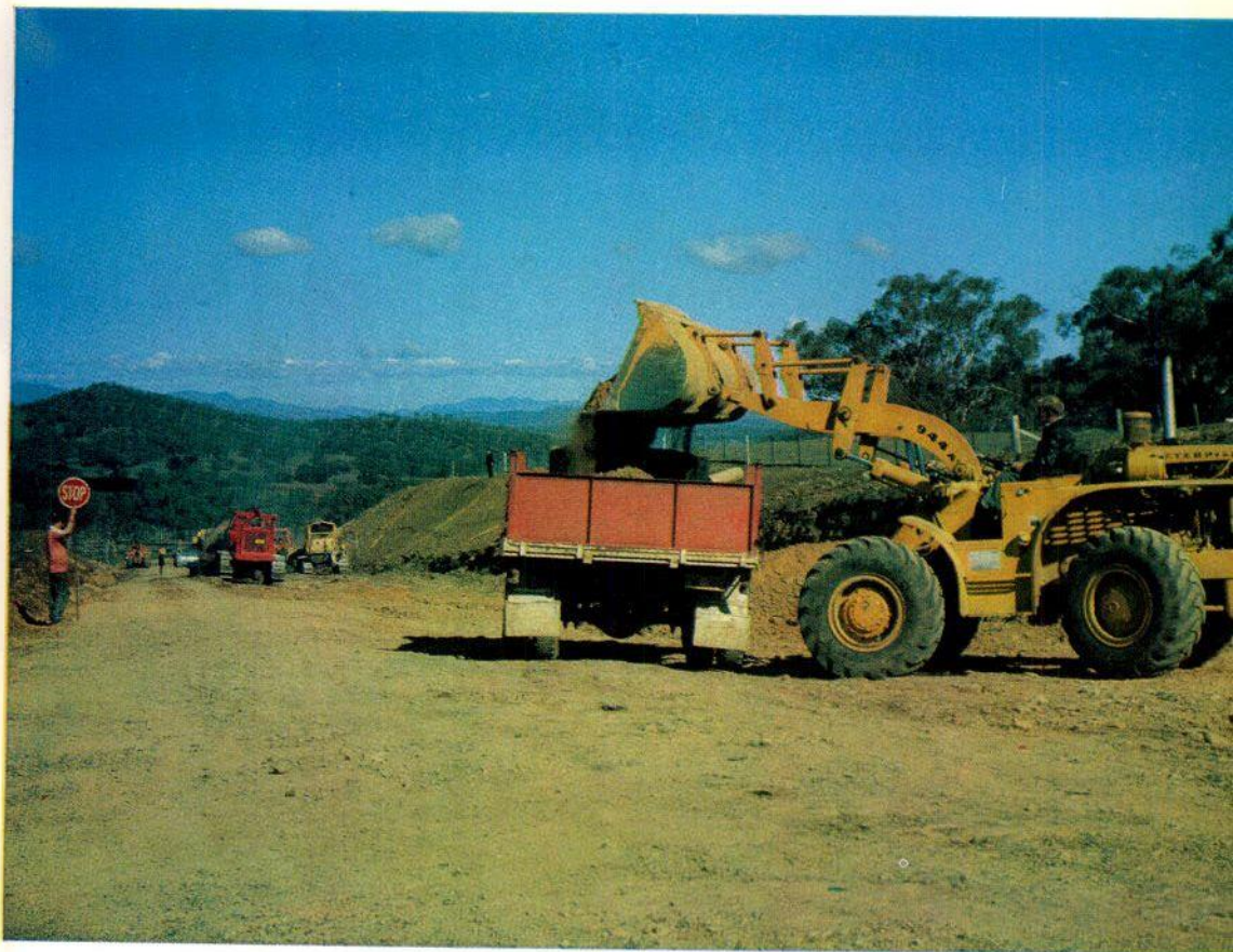
Reconstruction in progress preparatory to bitumen surfacing on the New England Highway (State Highway No. 9), 27 miles north of Murrurundi.
