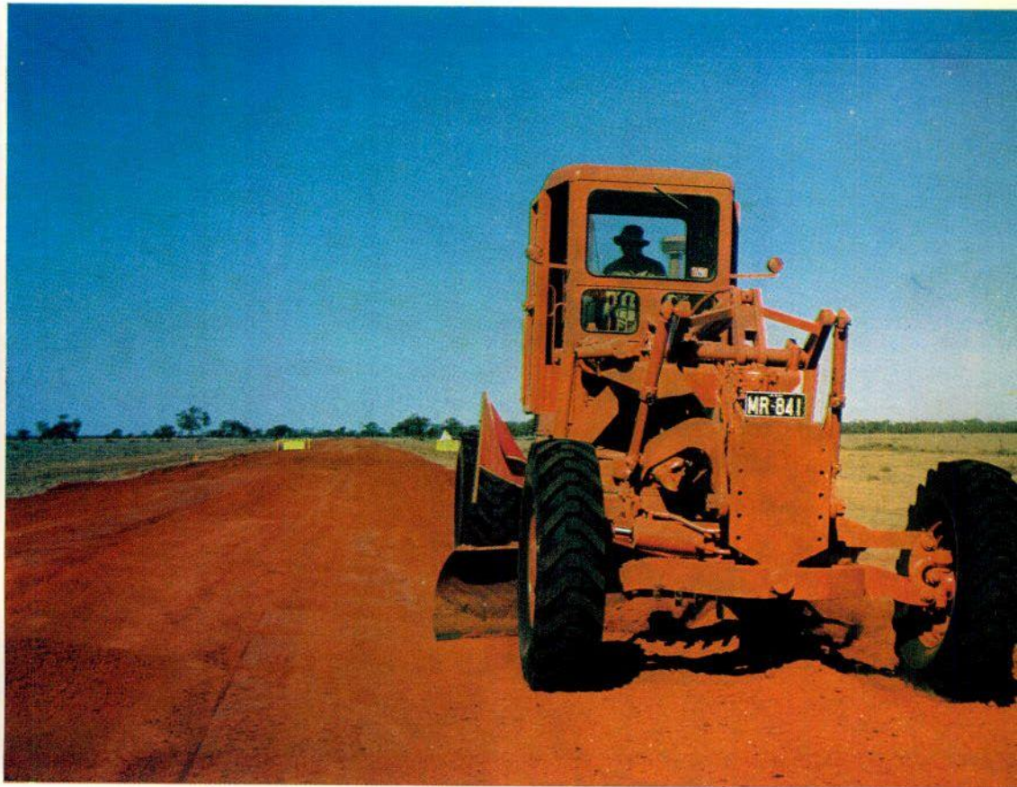
Reconstruction preparatory to bitumen surfacing on the Mitchell Highway (State Highway No. 7), 74 miles north of Bourke.
