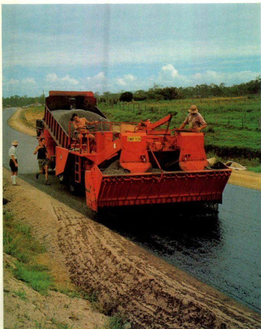
Laying aggregate on bitumen during the construction of a deviation of the New England Highway near Beresfield.
