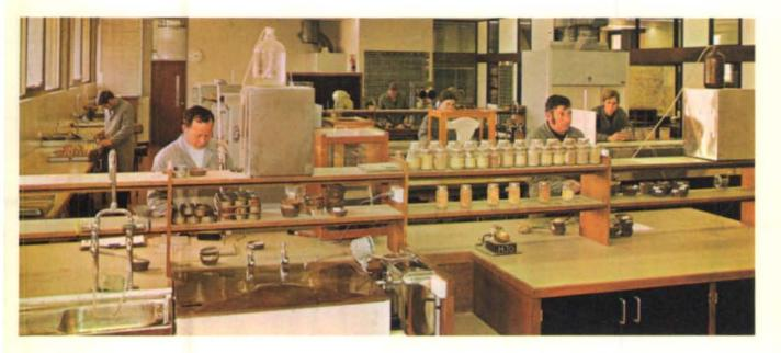
Above and right; The physical and chemical testing of materials, such as soils, gravel, aggregate and concrete, is carried out at a number of country centres, including the Department's new laboratory at Wagga Wagga. The laboratory is of contemporary architectural design and modern testing equipment and facilities are provided.
