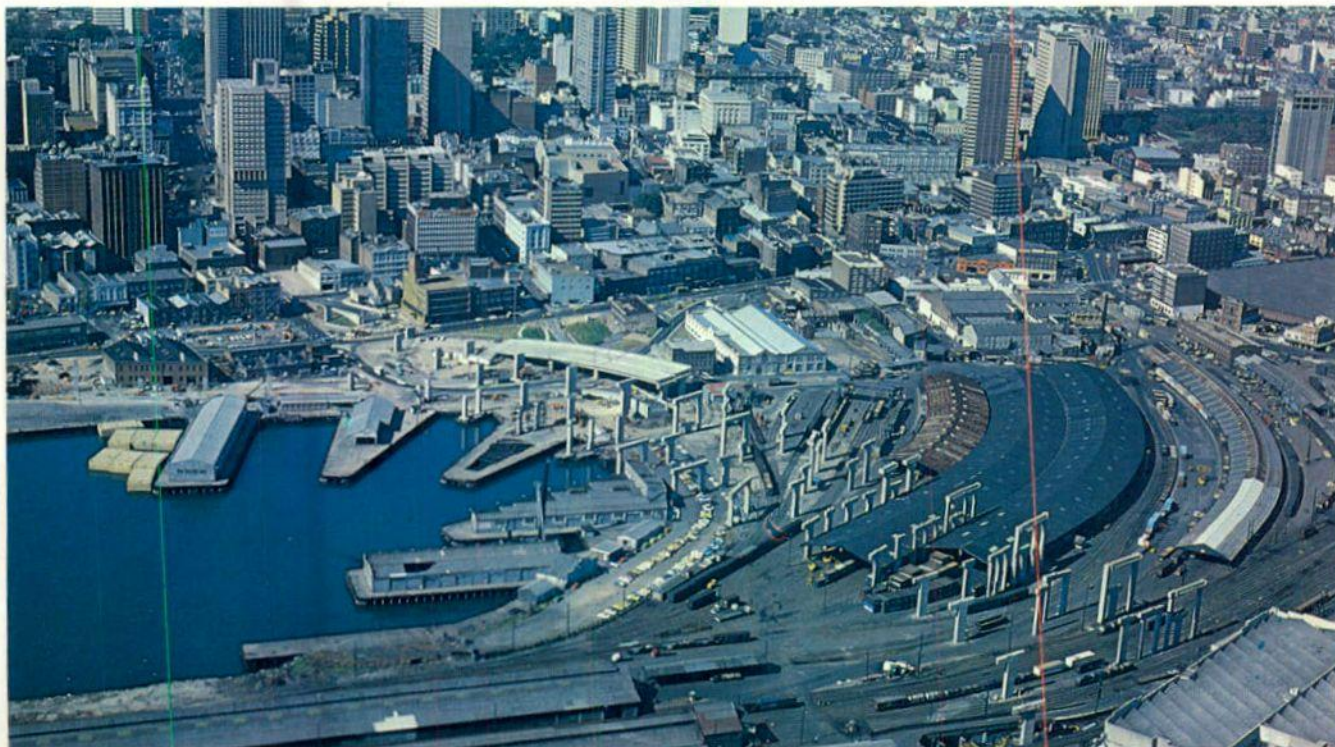
The viaduct on the North Western Freeway across Darling Harbour railway goods yard is taking shape with the construction of the deck.
