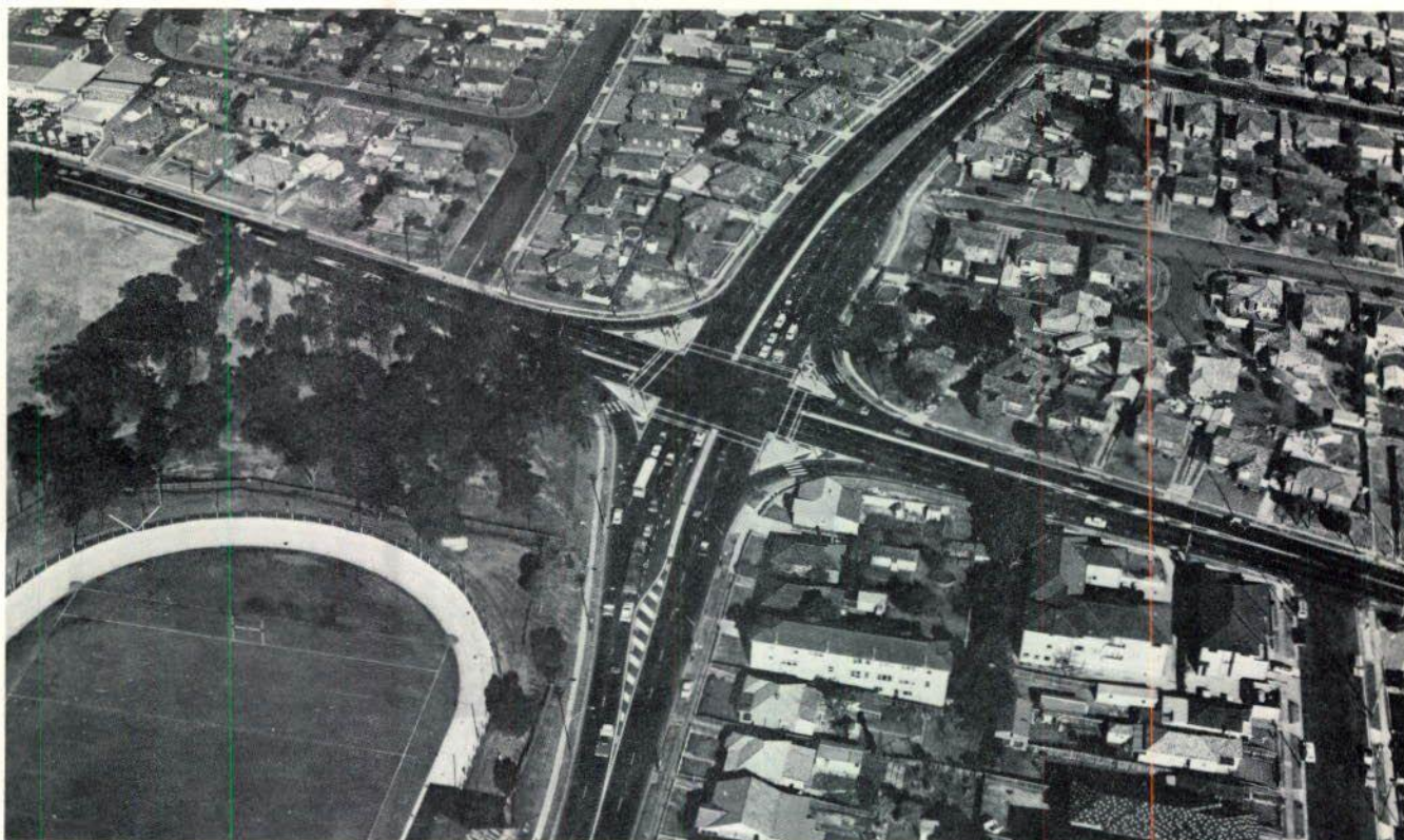
The recently reconstructed intersection of King Georges Road and Canterbury Road at Wiley Park provides greater traffic safety by the separation and channelisation of traffic lanes with medians, traffic islands, storage lanes and wide merging lanes.
