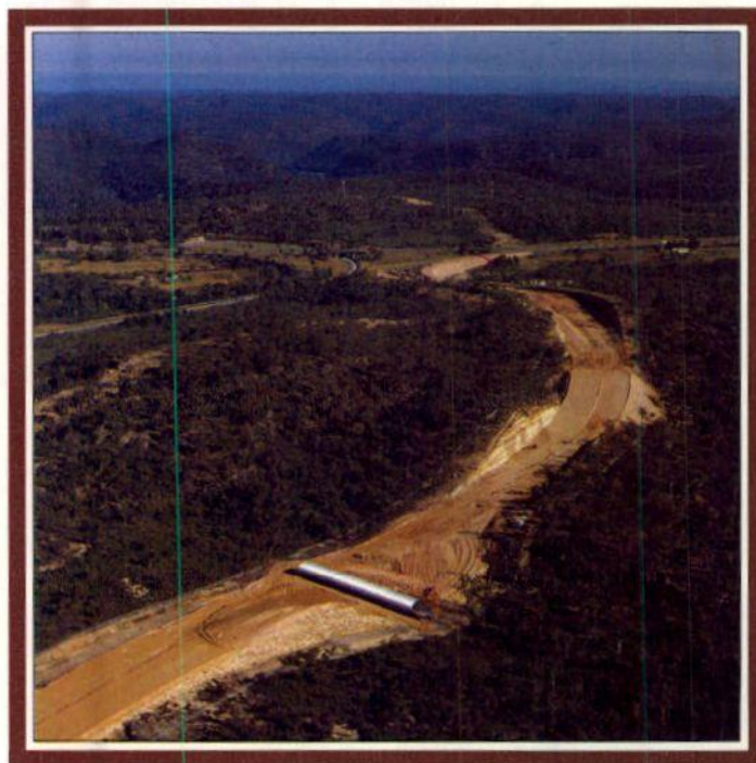
This steel underpass will allow both animals and pedestrians to cross the F3 — Sydney-Newcastle Freeway between Calga and Mooney Creek.
