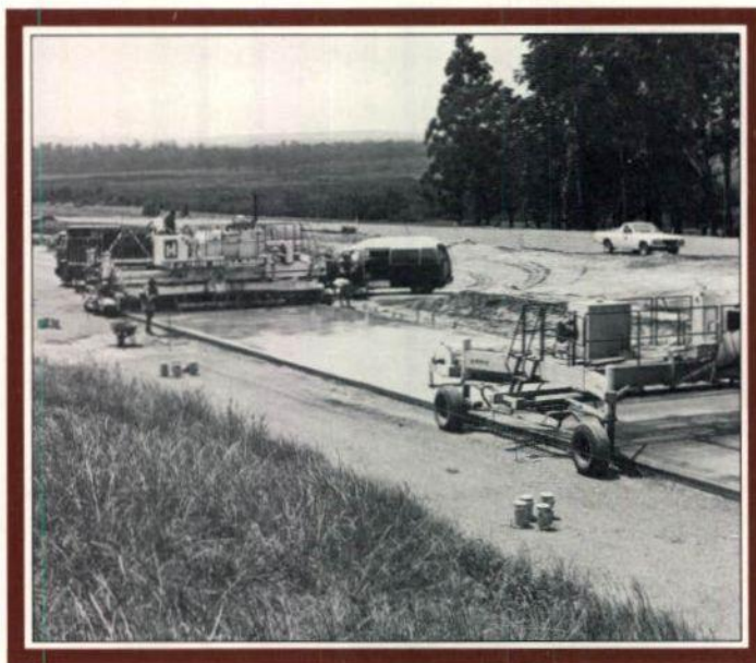
Unreinforced concrete pavement being laid by a slipform paving machine on the Wyong to Wallarah Creek section of the F3 — Sydney-Newcastle Freeway.
