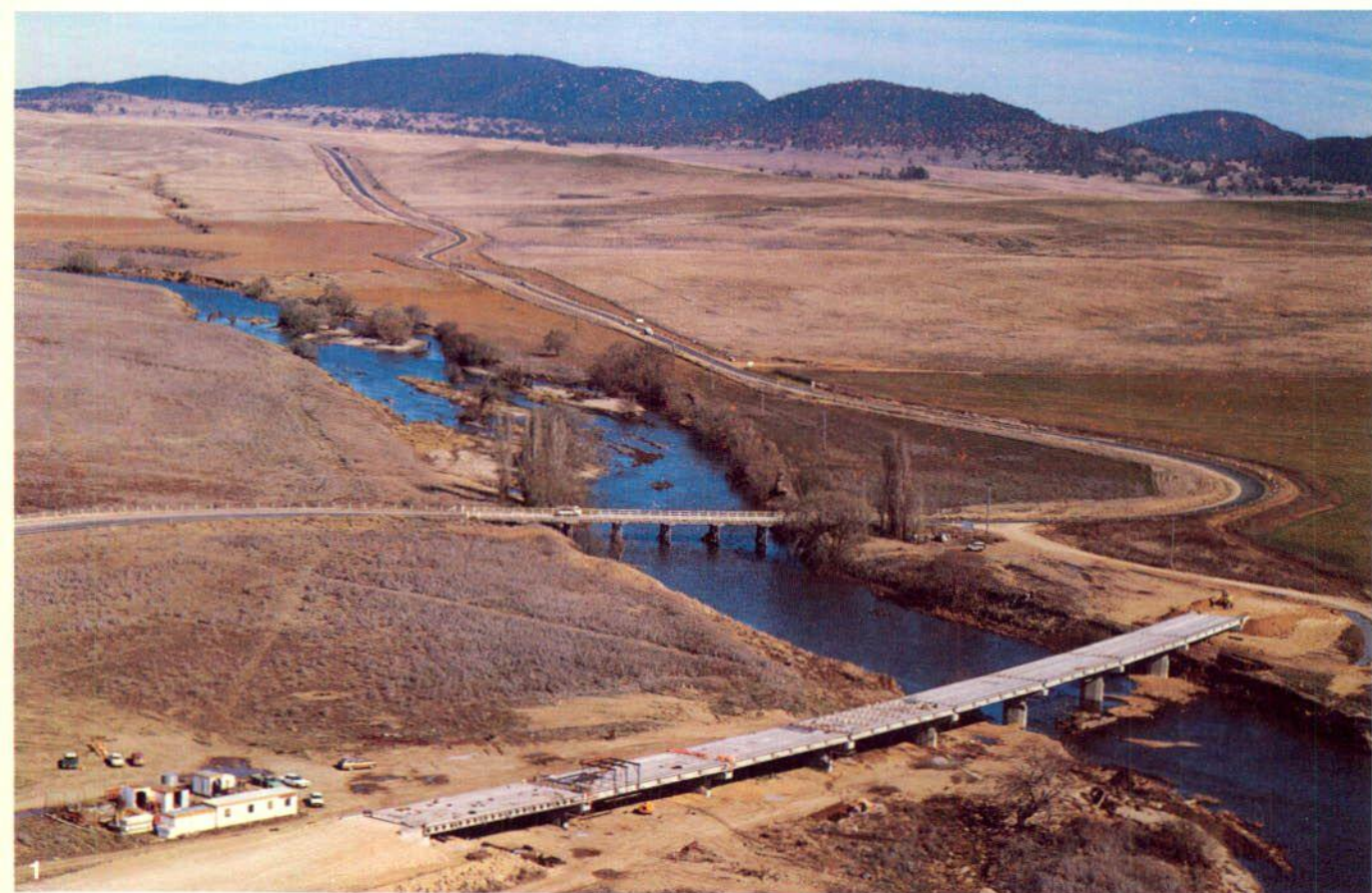
1. A new bridge over the Numeralla River (in the foreground) and another over the flood plain will provide a flood-free route for the Monaro Highway
