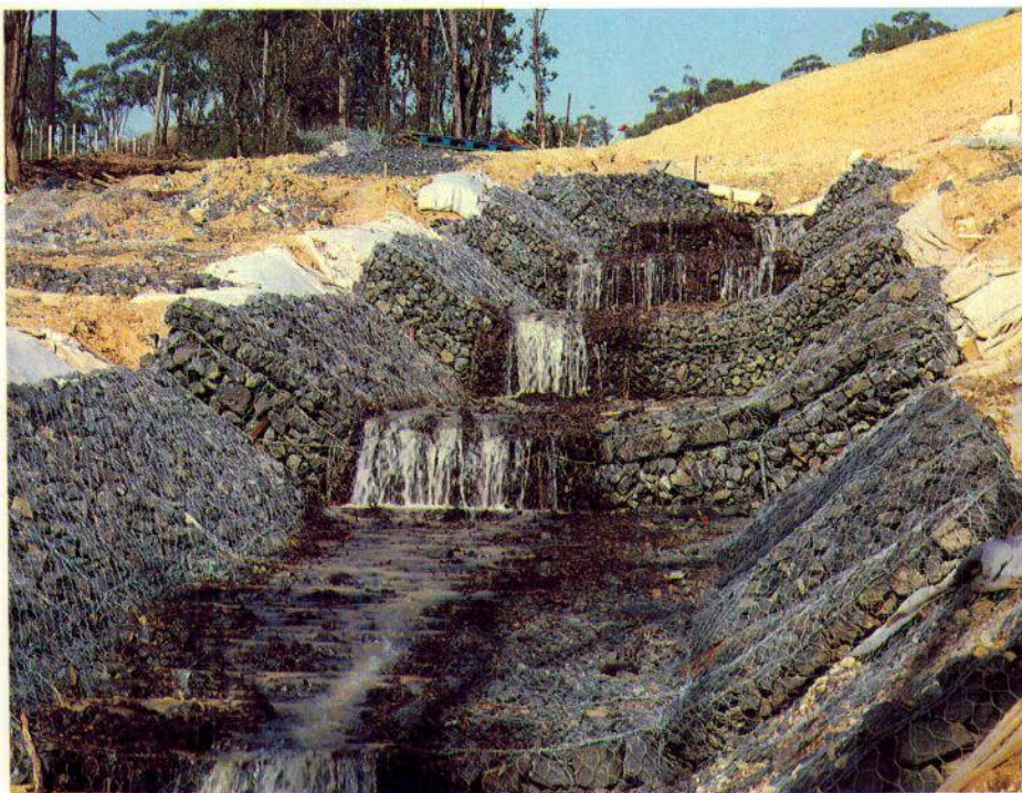
Erosion control along the F3 — Sydney-Newcastle Freeway using the Reno-Mattress method.
