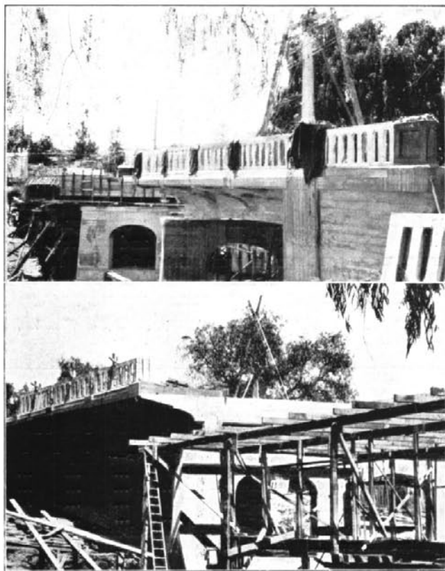
Reinforced concrete bridge under construction in Short-street, Young.
