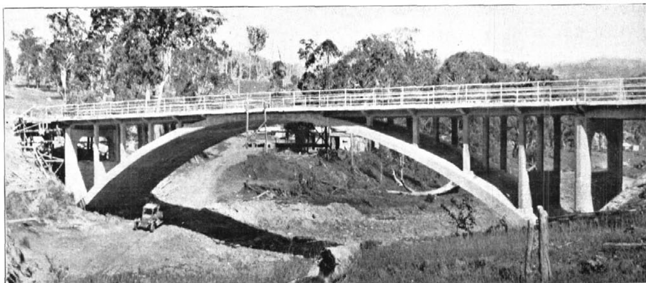
Completed 160 ft. reinforced concrete arch span, Koreelah Creek bridge, Great Northern Highway, Shire of Tenterfield.
