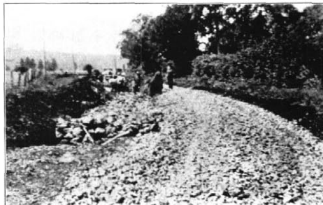
On the North Coast Highway at Cumbulum. Using fascines of mangrove bushes and spalls to prepare a road foundation on waterlogged clay.
