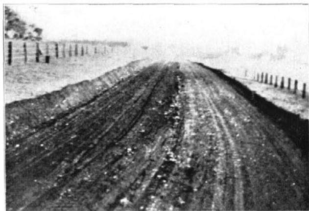
Formation built by tractor and grader only, without use of plough or scarifier.
