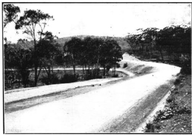
Cox's River Deviation, Gravel Pavement near Meadow Flat. The old road is shown at the left.
