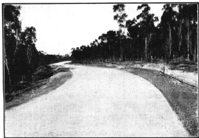
Cement Penetration Pavement. Cox's River Deviation.
