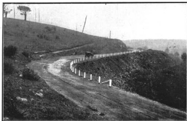
An example of difficult alignment on a main highway. The radius of the first curve is 150 feet, and of the second 200 feet, providing a sight distance of 180 feet.
