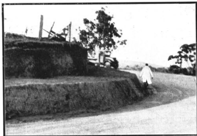
A curve of 100 feet radius. The sight distance has been increased by 50 per cent. (from 90 feet to 140 feet) by the benching shown.
