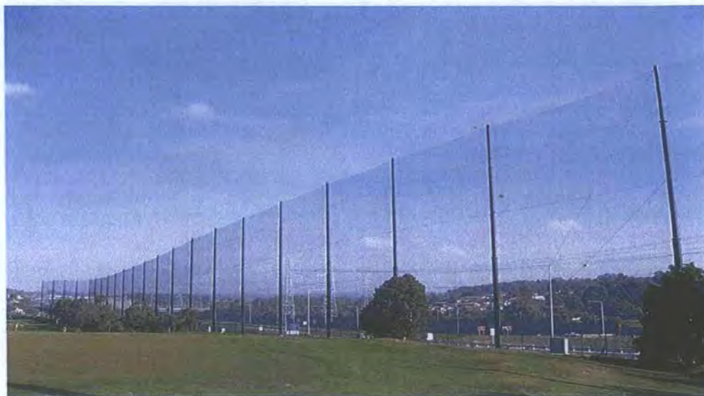
Ringwood Golf Club – Melbourne At 30m tall this is the highest engineered fence in Australasia
