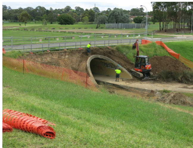
Hurricane Drive, Raby culvert corrosion repair
