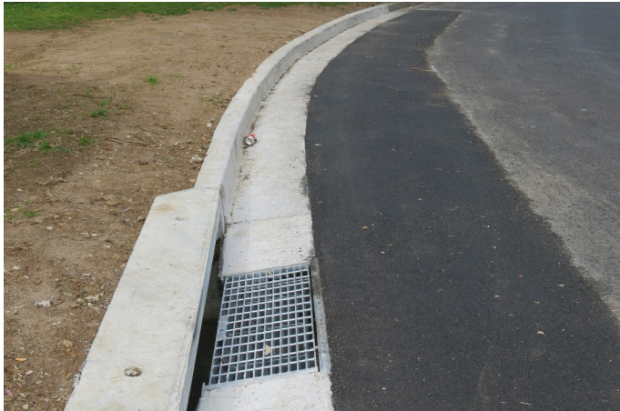
Damaged stormwater grate and kerb and gutter reconstruction at Canberra Crescent, Campbelltown
