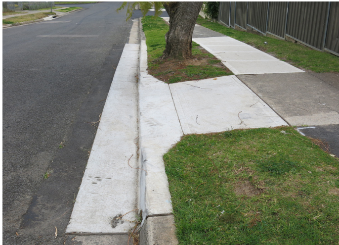
Kerb and gutter along with layback at Valley Road, Campbelltown
