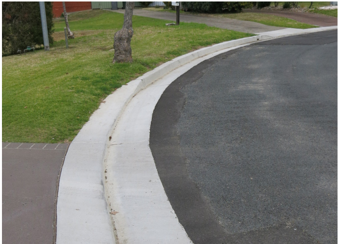
Kerb and gutter with layback replacement work at Colo Place, Campbelltown
