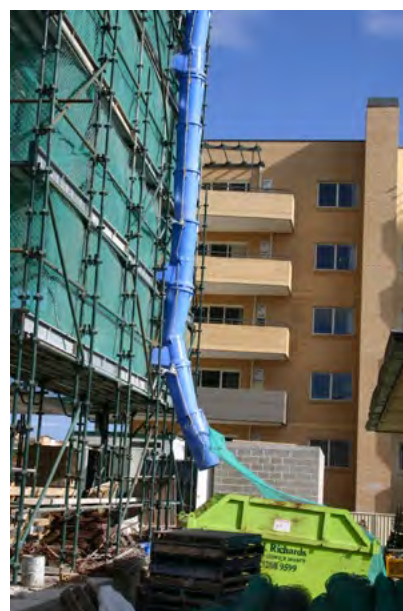
Figure 2.15.2 - Example of management of construction waste.
