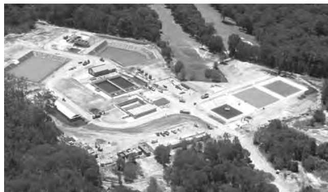
Woodford Island STP under construction
