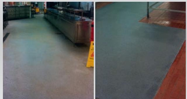
Industrial strength non slip coating applied over tiles in major hotel.
