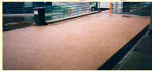
Industrial long lasting non slip application rendering a high coefficient of friction rating for pedestrian traffic and excellent non skid for vehicles and forklifts.
