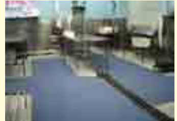
Cosmetically attractive and highly non slip coating applied in a constantly wet food preparation facility.
