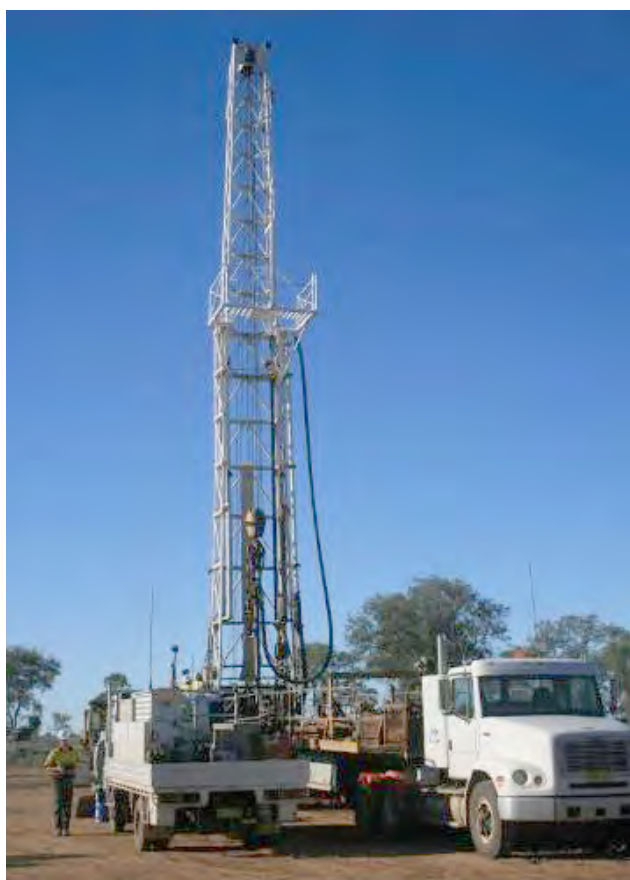
The department's drilling team sinking a new deep artesian bore at Polly Brewon homestead, north of Coonamble (Photo – NSW Office of Water)
