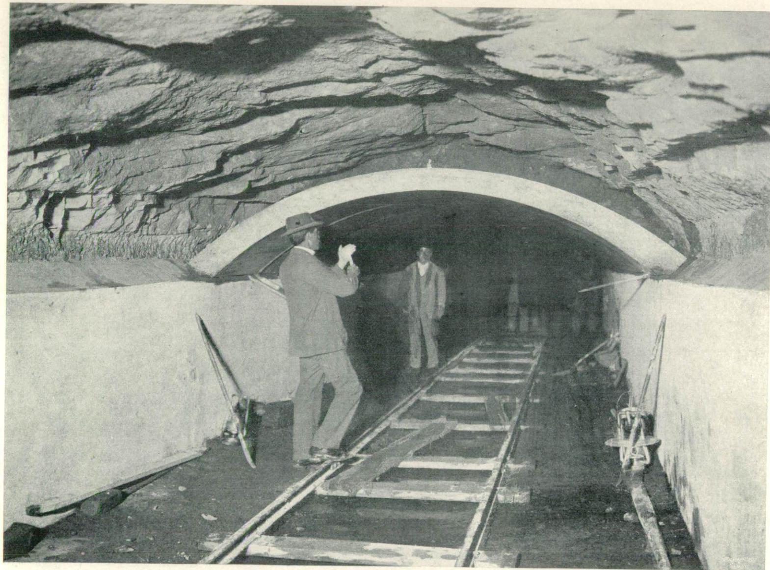
MARRICKVILLE STORM-WATER CHANNEL: TUNNEL WITH 'MONIER' ROOFING.
