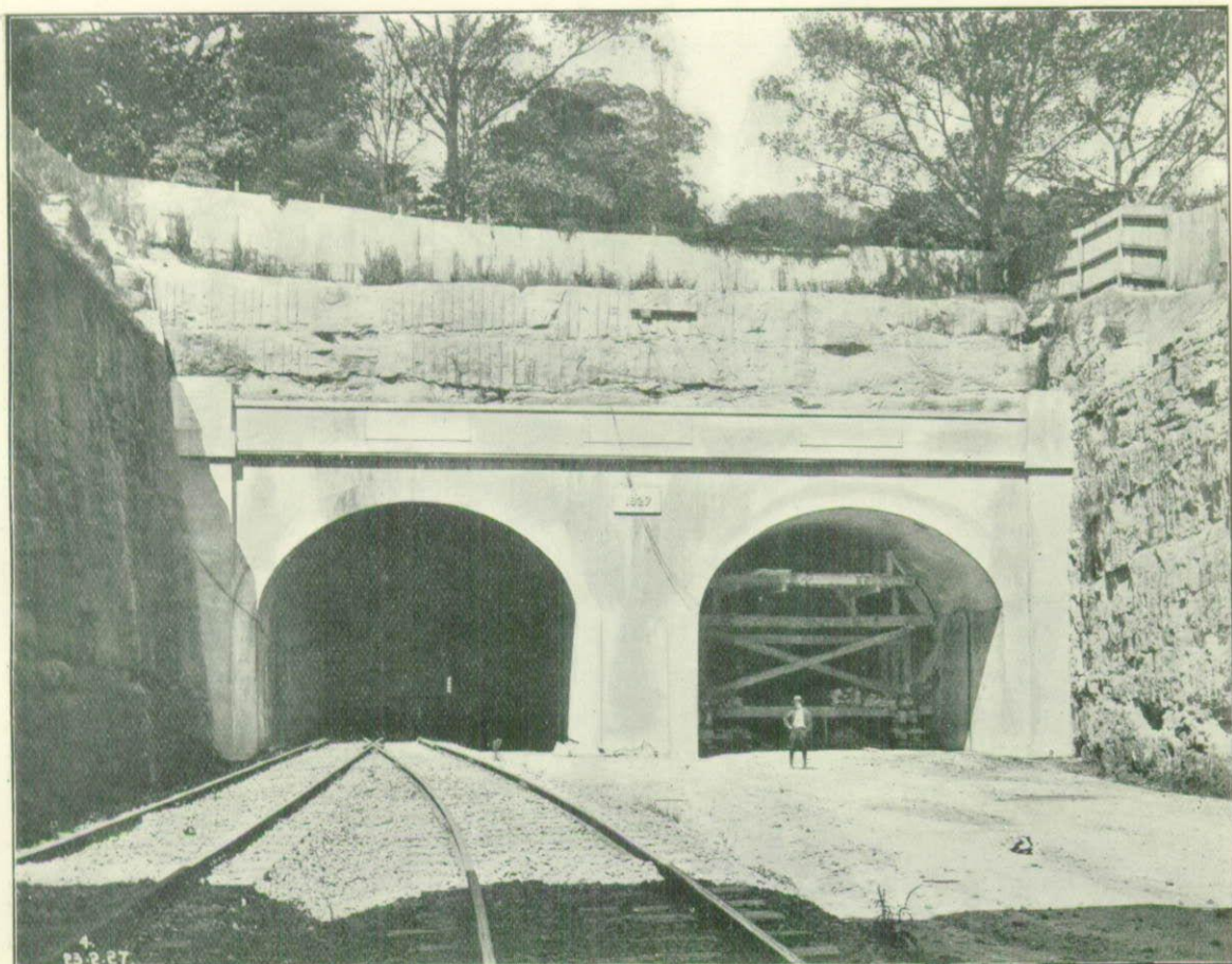
The portal near Bank-street for the Two Double Track Tunnels.
