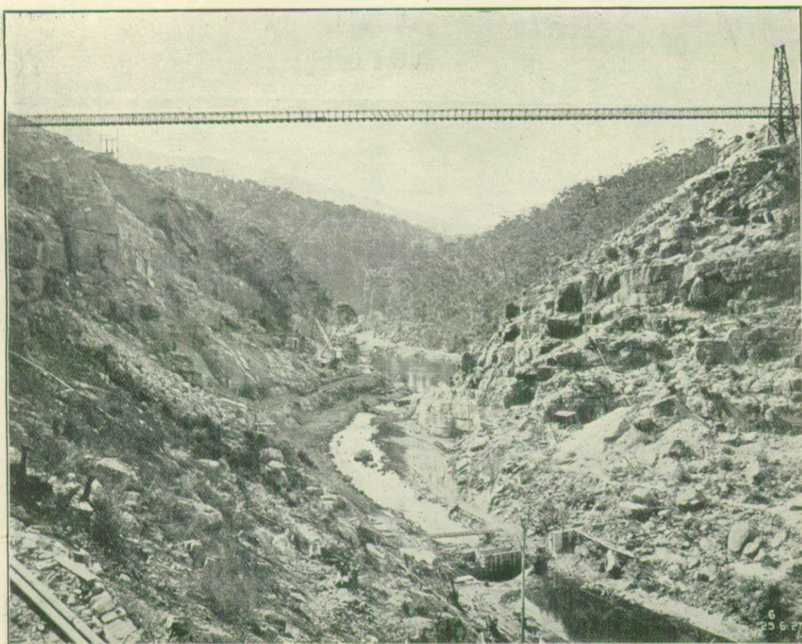
Nepean Reservoir : General view of Dam site showing suspension bridge, upstream diversion wall, and excavation for foundations.
