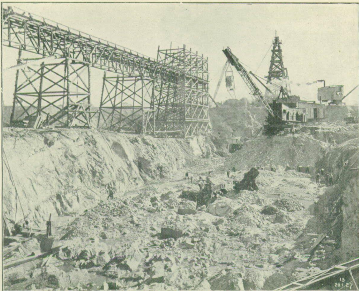
Hume Reservoir : View showing excavations for foundations for Spillway and South Wing Wall ; also trestle supports for Concrete Belt Conveyer.
