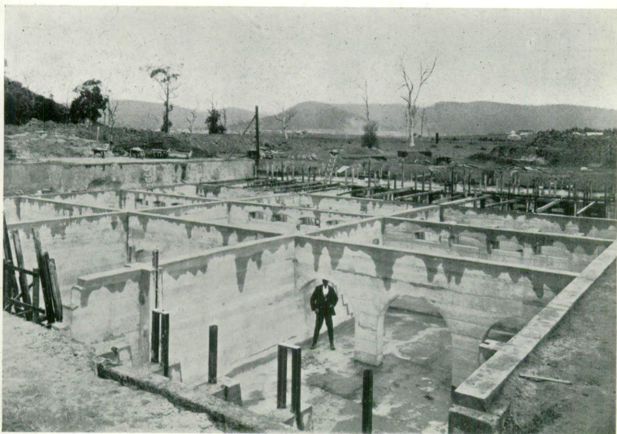
LITHGOW SEWERAGE.—SEPTIC TANKS BEFORE ROOFING.
