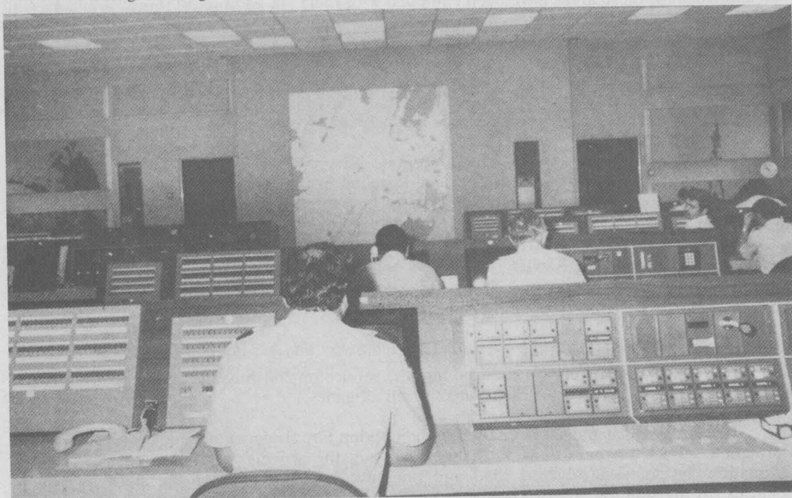
Fire alarm data is fed into a computer by a keyboard on one of the numerous consoles in the Centre and is shown on the visual display units and from a print-out complex
