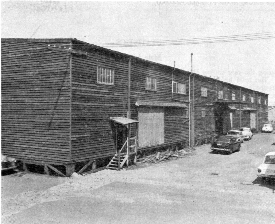
Exterior of Shed 66, Shea's Creek, which will provide additional Repository accommodation. The unpainted weatherboard construction of the shed may be clearly seen.
