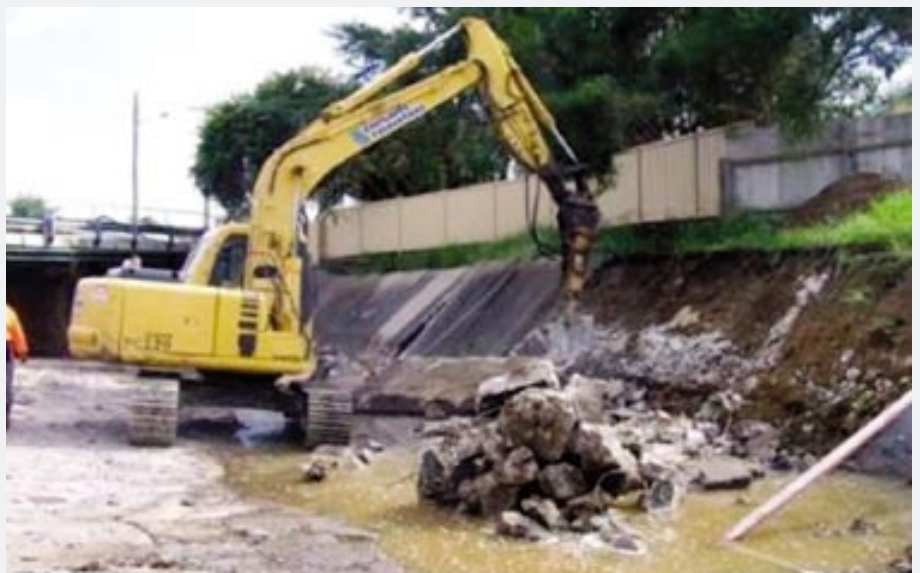
Repair of Cessnock Stormwater Channel
