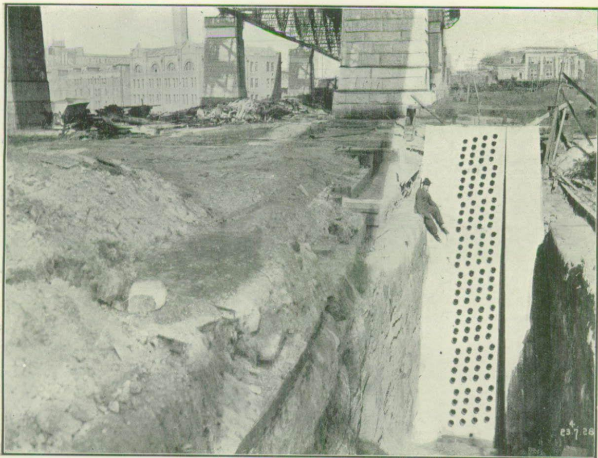
The Tunnel Cable Saddle; each pipe is 4\frac{1}{2} -inch diameter and will take one anchorage cable. There are 128 cables in all, 3-inch diameter.
