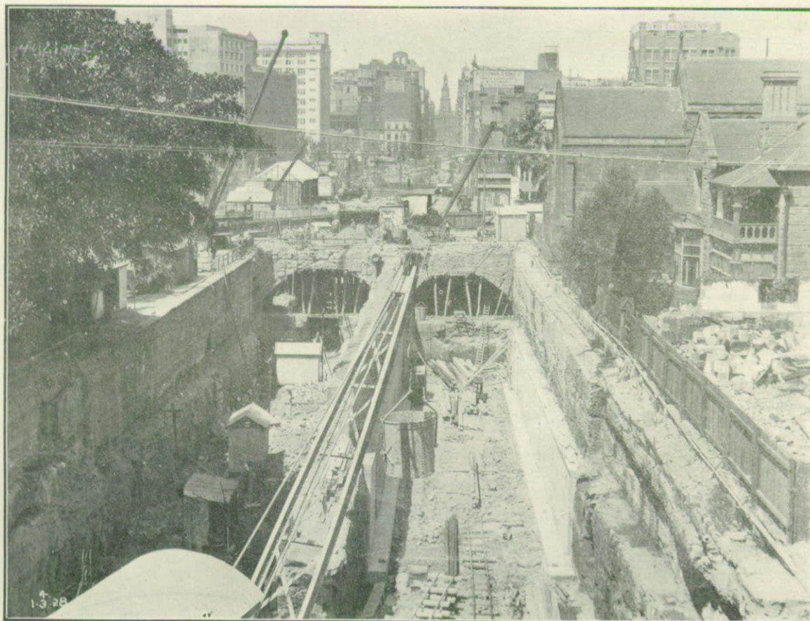
The double track construction, providing for four railway tracks under York-street.
