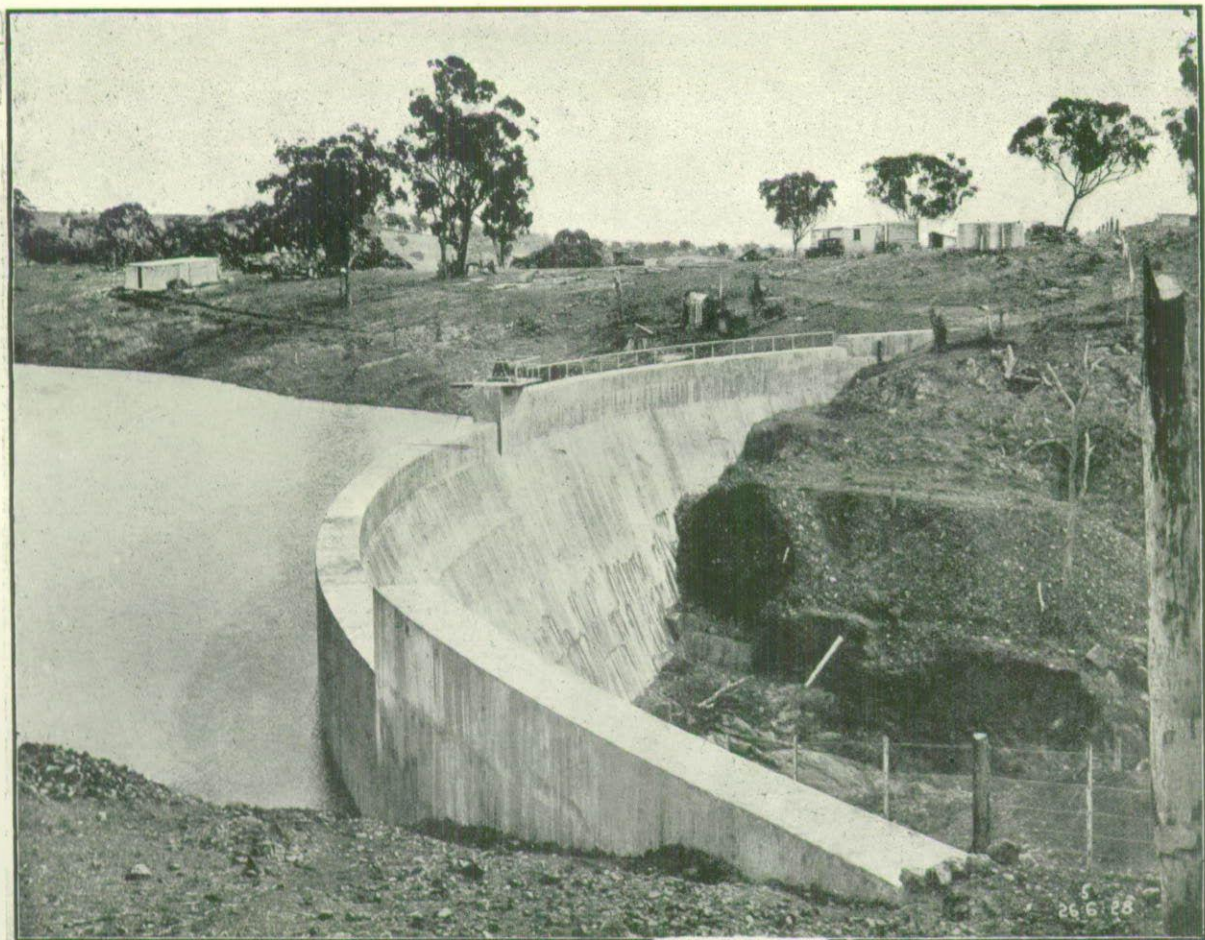
Molong Water Supply Dam built across Borenore Creek from which the water gravitates to a service reservoir in Molong. The capacity of this dam is 67,000,000 gallons.
