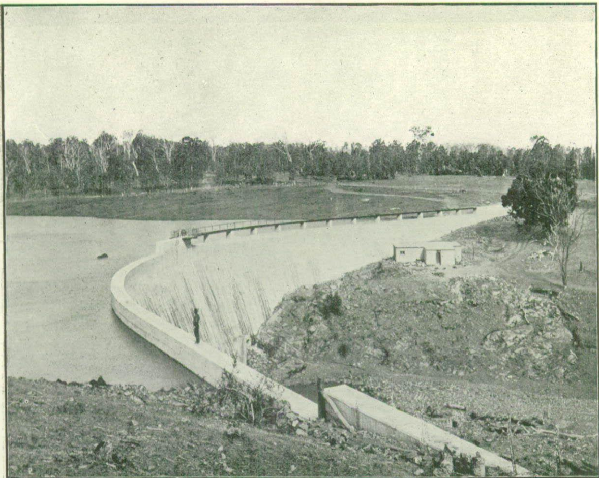
Armidale Water Supply Storage Dam built across Puddledock Creek from which the water gravitates to service reservoirs in the town. The capacity of this dam is 206,000,000 gallons.
