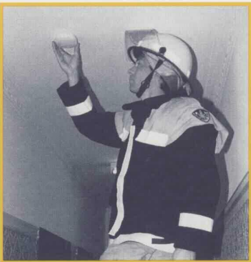
Firefighter Steve Yew from Randwick Fire Station installing a smoke alarm
