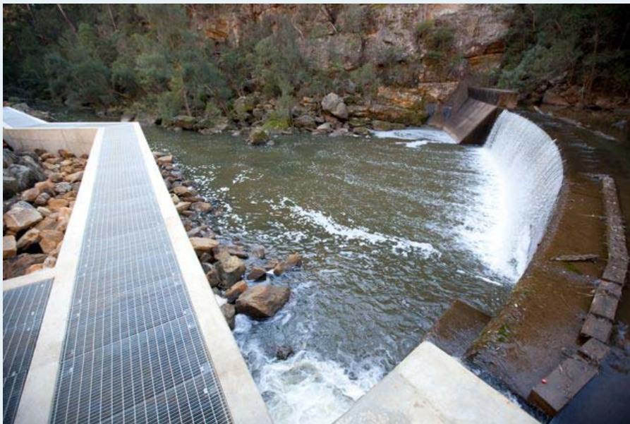
Caption: Theresa Park Weir was one of 10 along the Nepean River to have a new or upgraded vertical slot fishway installed.
