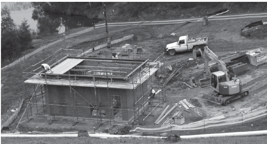
Work under way on the new raw water pumping station to access deep water in Upper Cascade Dam, in the Blue Mountains
